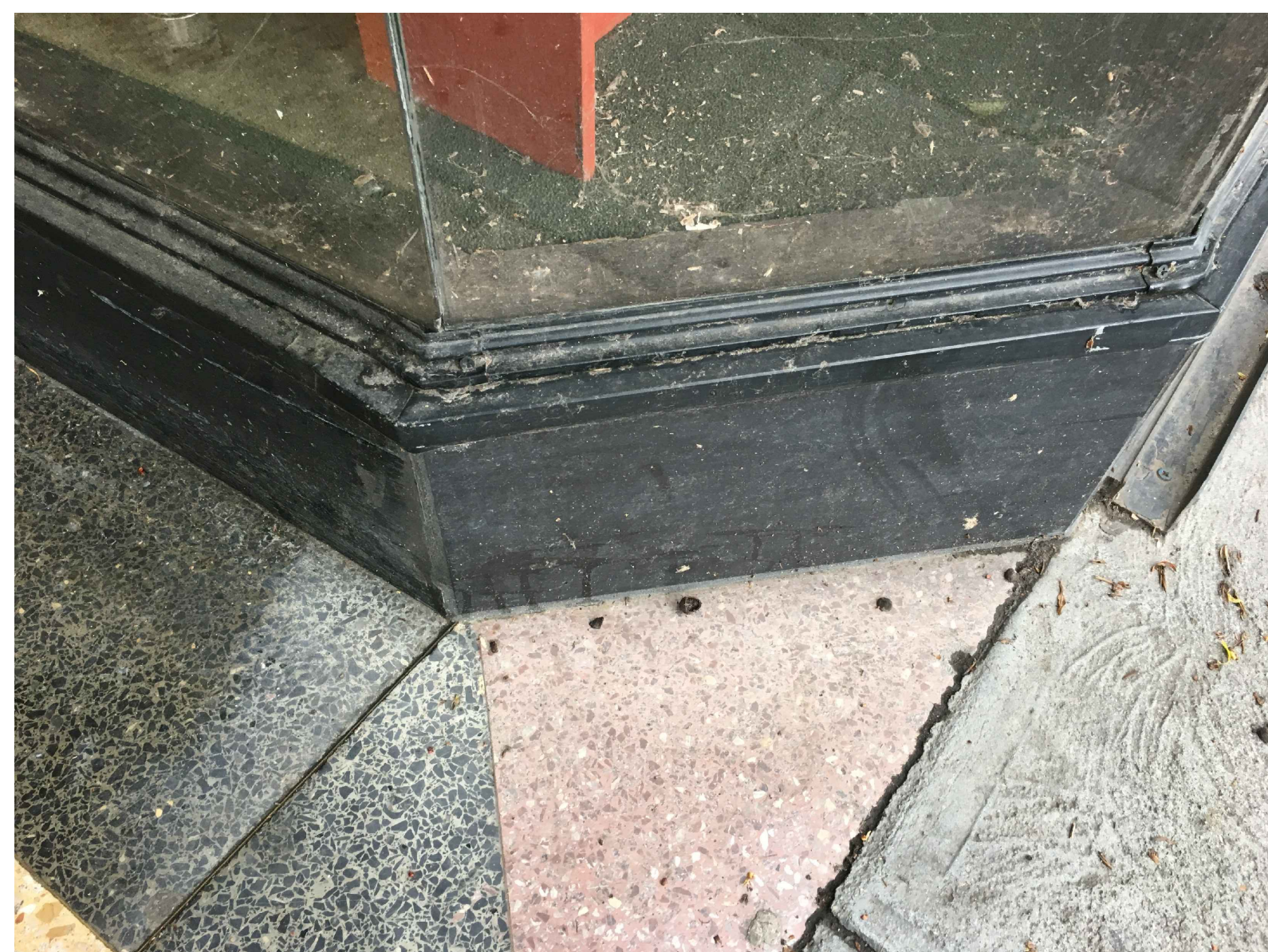
EXISTING METAL STOREFRONT AND CURB
